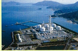
[ new Unit2 at Yanai Power Station ]
